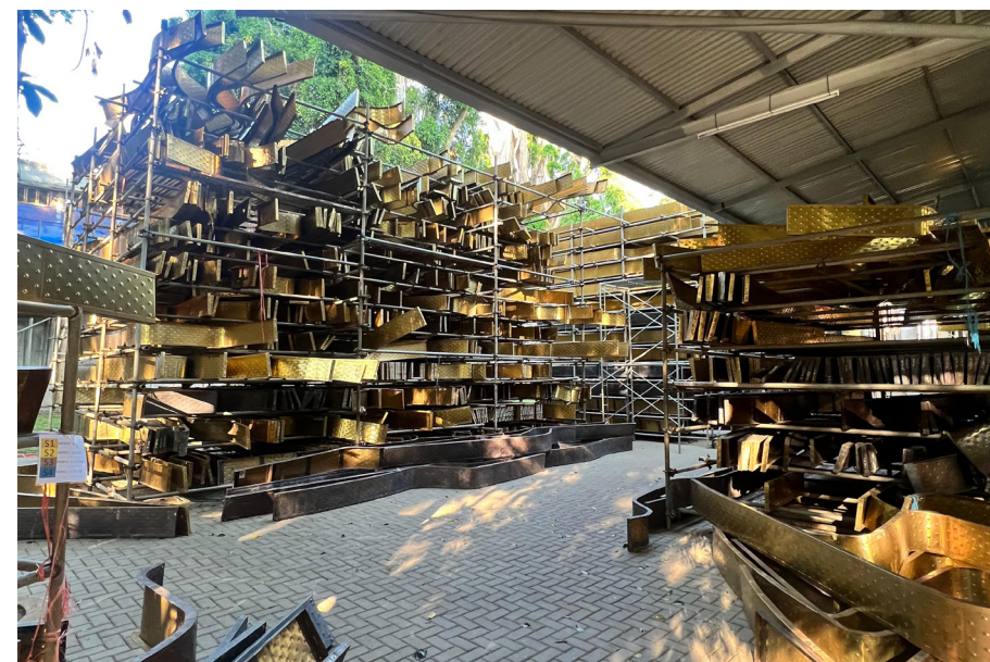
The building at 25% of the construction phase
